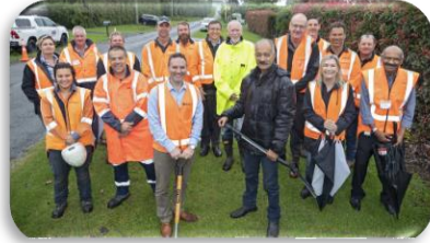
Mayor James Denyer and Pirirakau hapū kaumatua Peter Borell turn the first sod on the Prole Road project. Also pictured are Higgins construction crew, Western Bay councillors, staff and project consultants.
