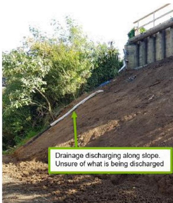
Figure 60: Existing drainage pipe on slope
