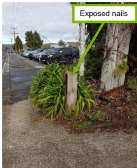
Figure 49: Exposed nails to the north of Te Puna School
