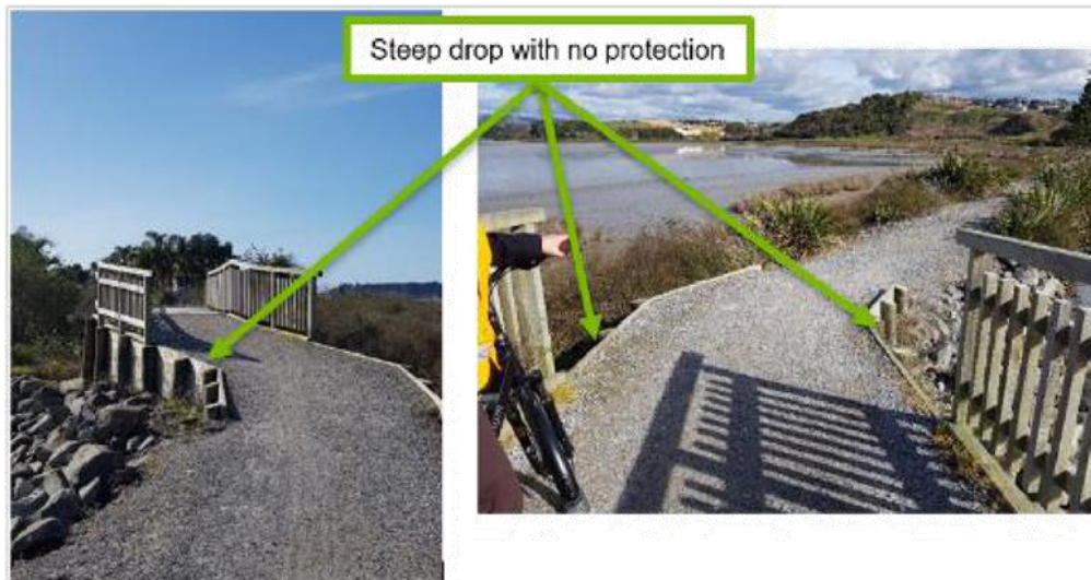
Figure 24: Wooden bridge with steep drop off at boardwalk
