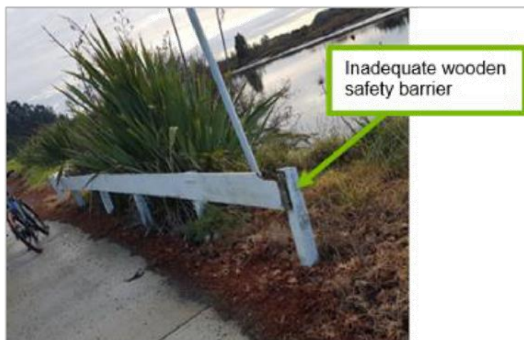
Figure 9: Inadequate wooden sight rail
