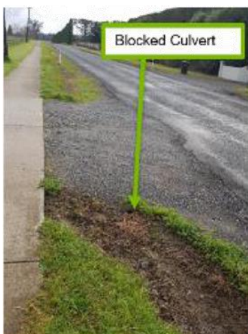
Figure 48: Blocked culverts along Te Puna Road
