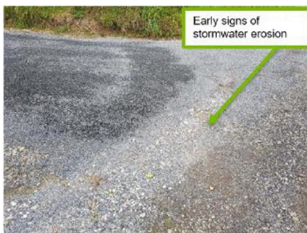
Figure 37: Signs of stormwater erosion
