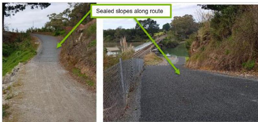
Figure 35: Loose chip on sealed surface at steep slopes
