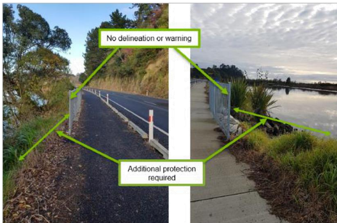
Figure 8: Barriers lacking warning strips and adequate delineation and inadequate drop off protection
