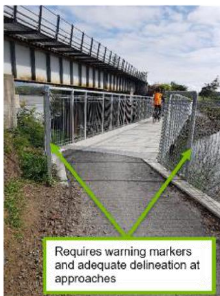
Figure 21: Bridge railing without adequate hazard markings
