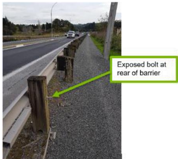
Figure 44: Snagging hazard Wairoa River bridge guardrail
