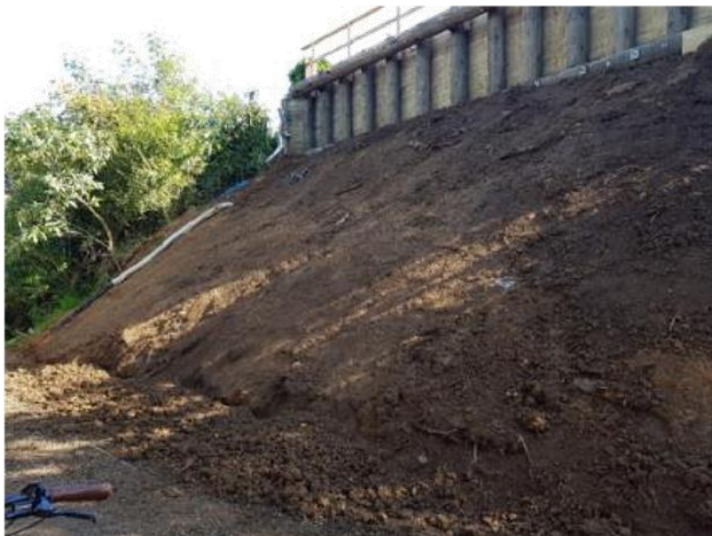
Figure 59: Existing slope which requires protection to avoid erosions and debris affecting the cycle path below
