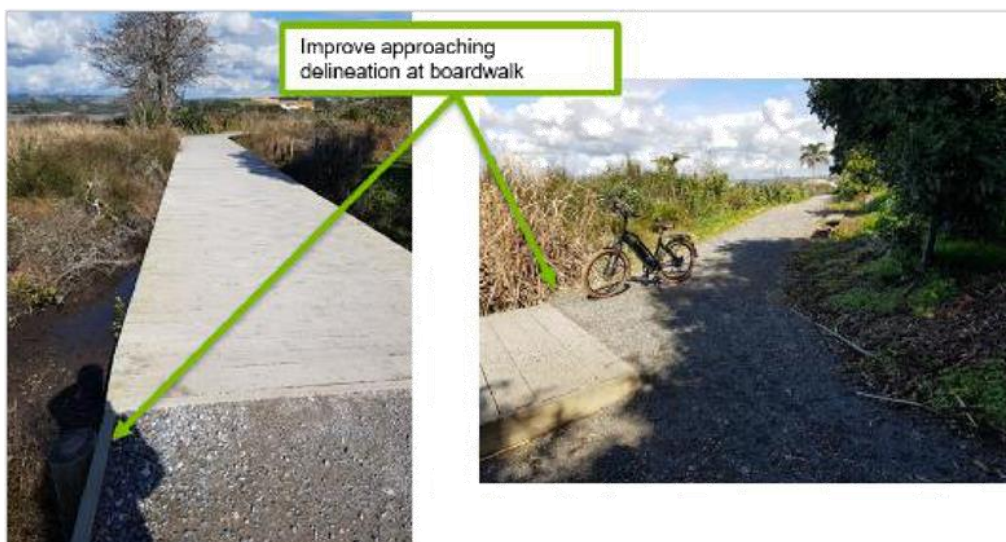
Figure 39: Boardwalk approaches without adequate delineation or warning
