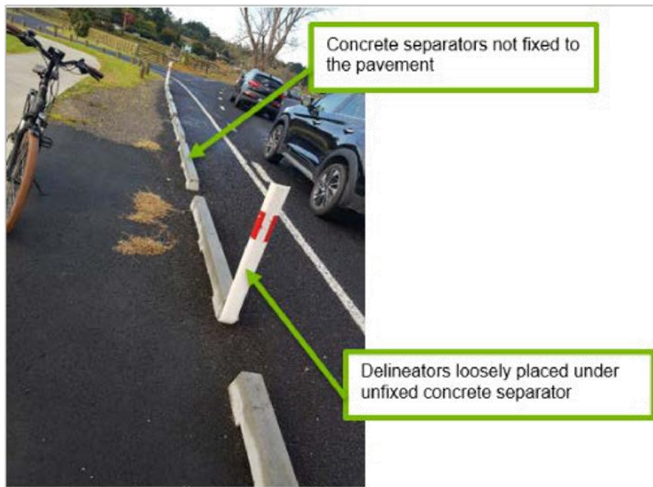
Figure 7: Concrete barrier not fixed on Te Puna Station Road
