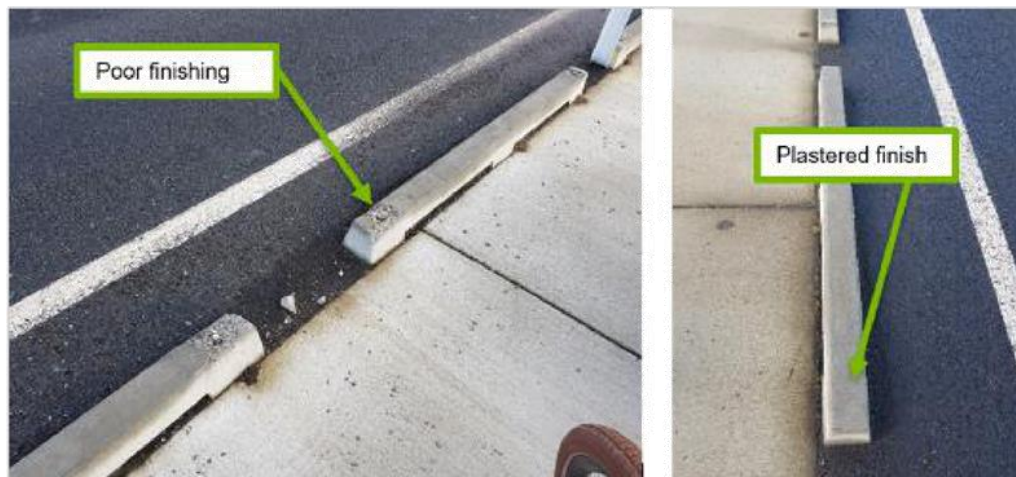
Figure 45: Poor finishing on concrete barriers along Te Puna Station Road
