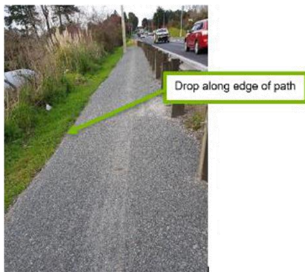
Figure 43: Drop along edge of path between SH2 and Wairoa Bridge
