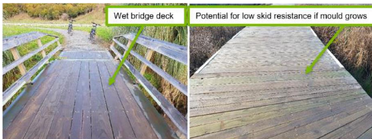
Figure 23: Wet bridge deck and possible mould growth
