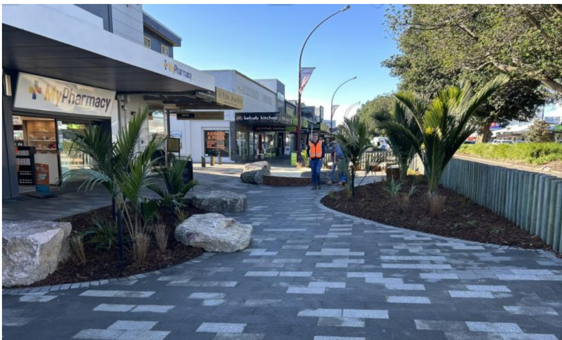
Figure 1: Completed Heritage Plaza Stage 1
