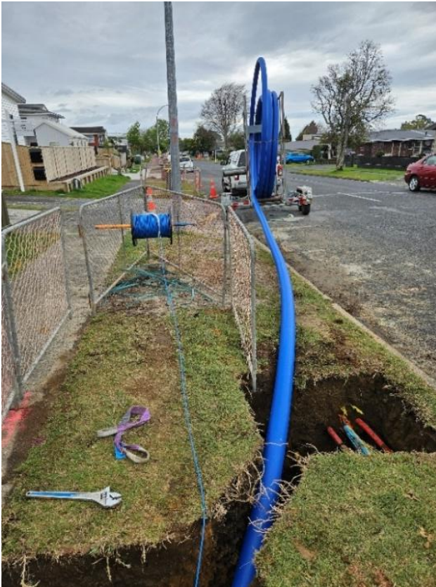
Installation of new 100mm pipe.
