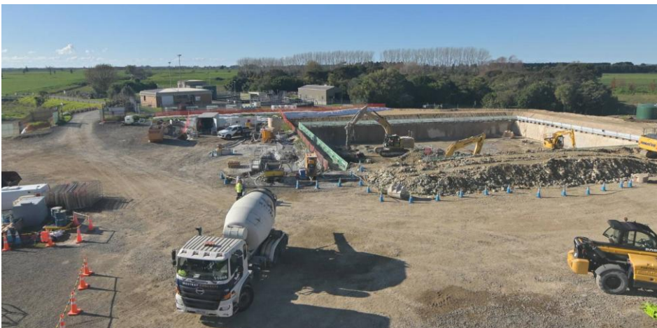
Gordon Street Wastewater Treatment Plant – Construction Progress 14 May 2026.
