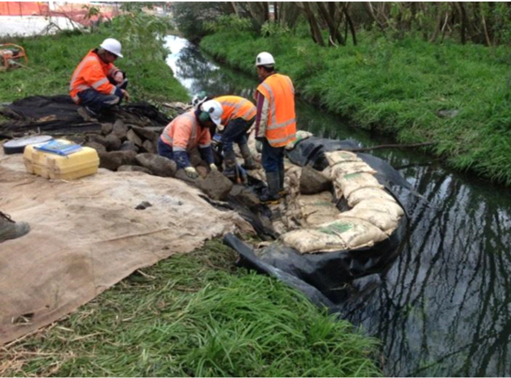
Figure 2b - Sandbag cofferdam example Photo credit: https://escanterbury.co.nz/project/diversions-task/
