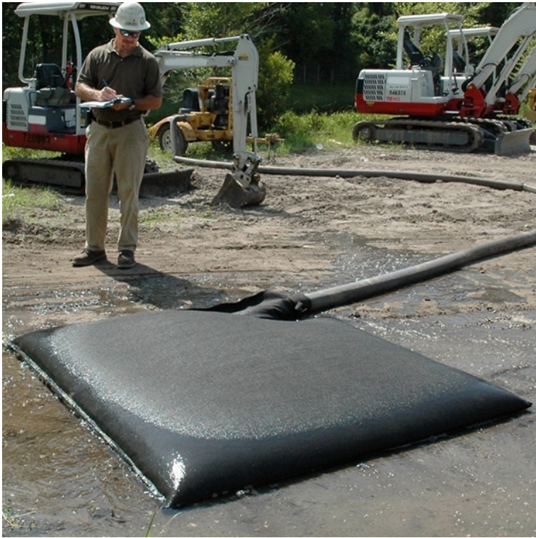
Figure 1b - Geotextile bag example. Photo credit: https://ph7.co.nz/products/ultra-dewatering-bag-4247/
