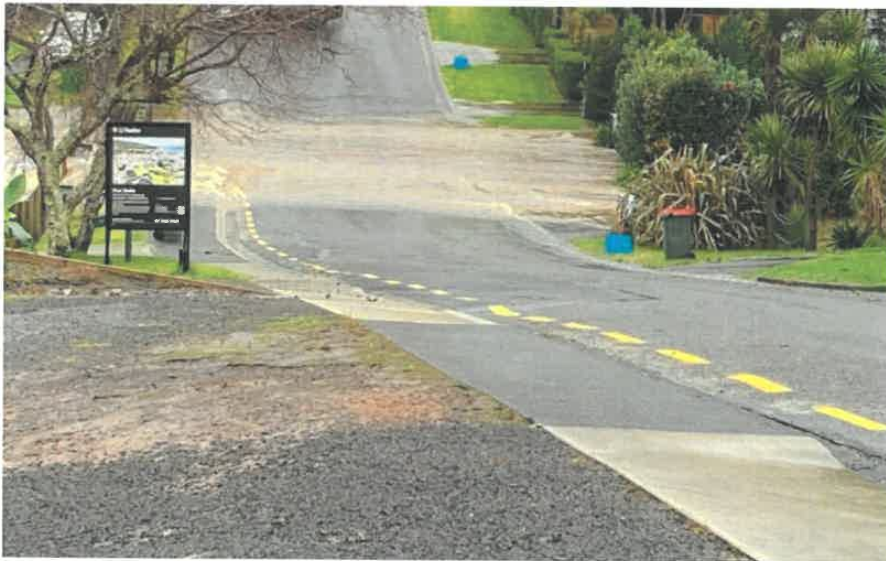
WATER FLOWING INTO PENSIONER FLATS FROM JENKINSON STREET LANE- 29 MAY
