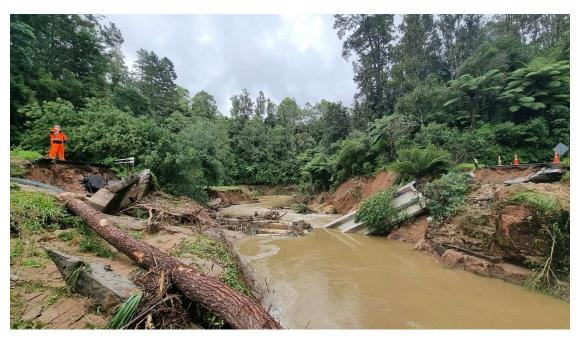
Figure 2: Photo of the existing bridge in the stream bed after the storm event, January 2023. The temporary road bridge occupies the location of the former double span concrete T bridge.
