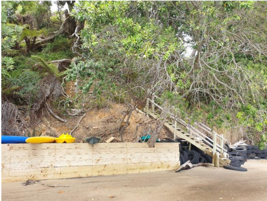
Photograph 3.3: Timber structure recently constructed at base of landslip (24/02/2021).
