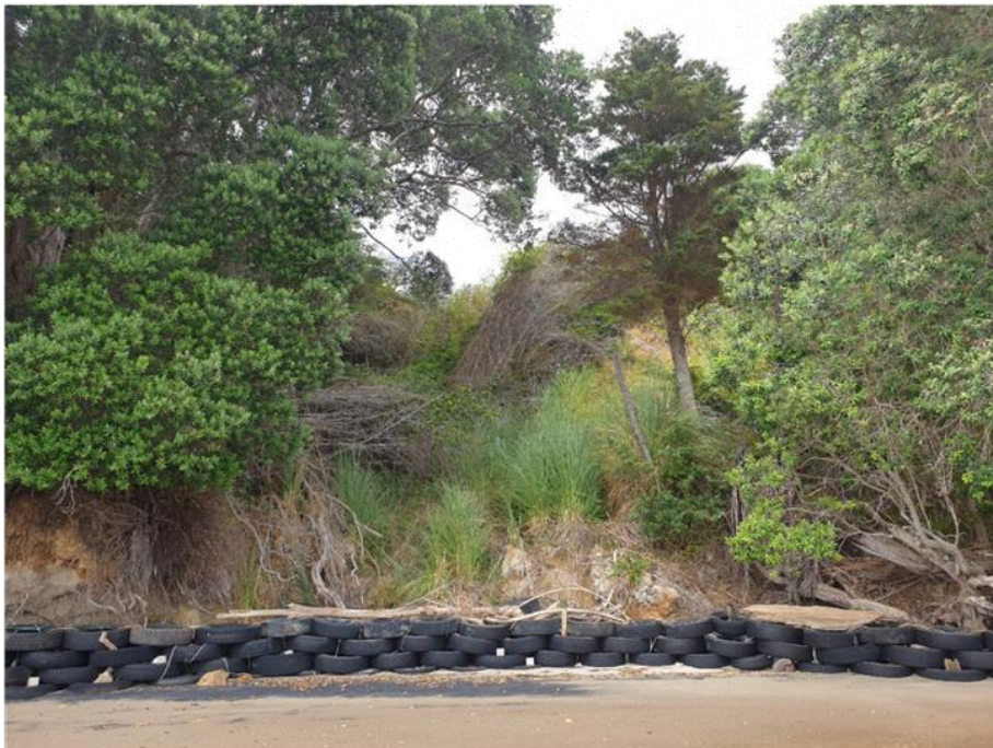
Photograph 3.2: Recently constructed tire wall along base of Landslip 7 (24/02/2021).
