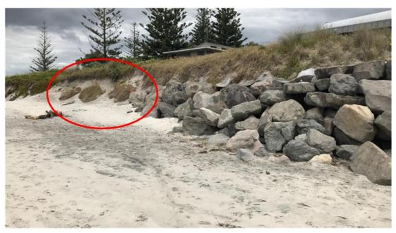
Figure 14b - Southern Termination of the Southern Seawall (red circle indicates more significant end effect erosion)
