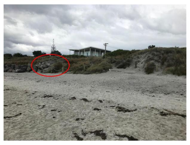
Figure 13a - Northern Termination of the Southern Seawall (red circle shows minor end effect erosion)
