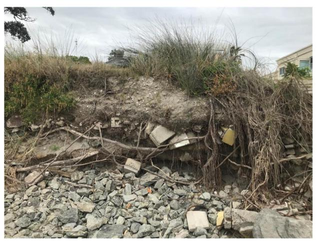
Figure 6 - Vertical bank littered with buried construction debris (Section A-A)
