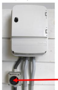
The panel must be mounted at an appropriate height to enable the service technician easy access in the event of a service issue.
